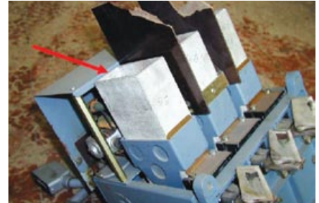
Figure 49 Electrical switchgear with asbestos flash protection
