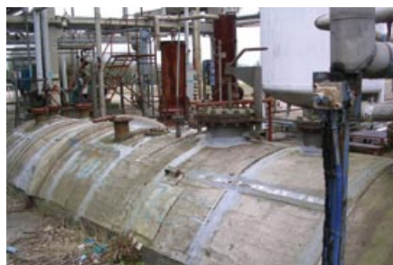
Figure 12 Lagging on large petrochemical vessel
