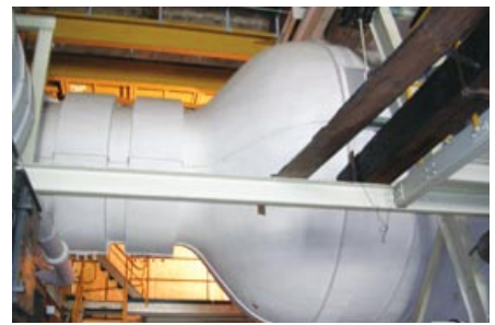
Figure 51 Vessel clad in amosite insulation
