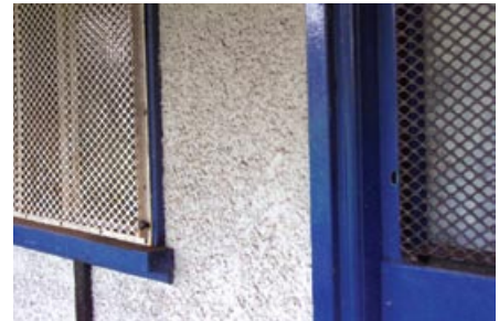
Figure 33 Chrysotile pebble-dash exterior wall coating
