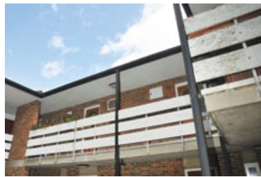
Figure 18 AIB exterior panel on open walkway
