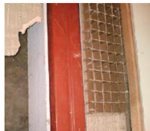
Figure 21 AIB column fire protection in CLASP building
