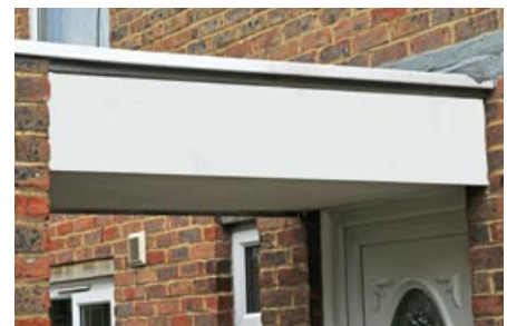
Figure 15 AIB panel in porch
