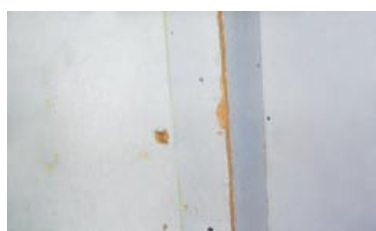
Figure 24 Chrysotile paper on fibreboard boxing
