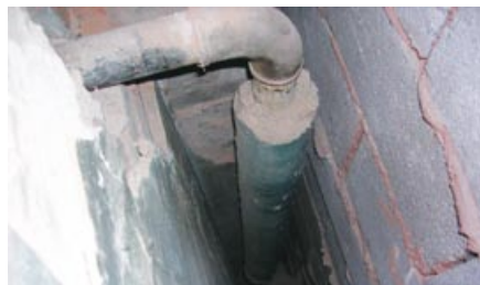
Figure 9 Lagged pipe in wall cavity
